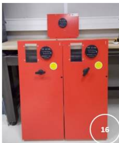
Stick of self-adhesive supports of cover with instructions next to each porthole.
