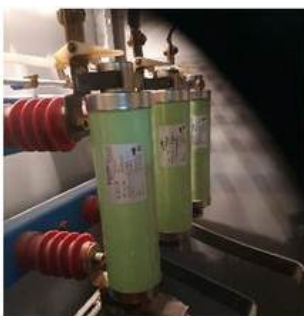
Through a window H.VIR
