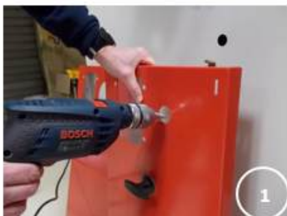
With E. Robur drilling tool, drill a hole of \varnothing 10 mm.
